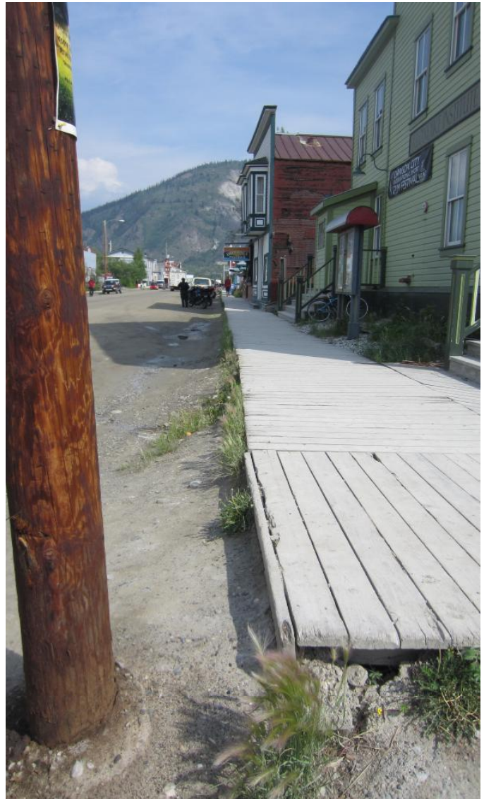
Inaccessible Boardwalk at the corner of Princess Street and Second Avenue
