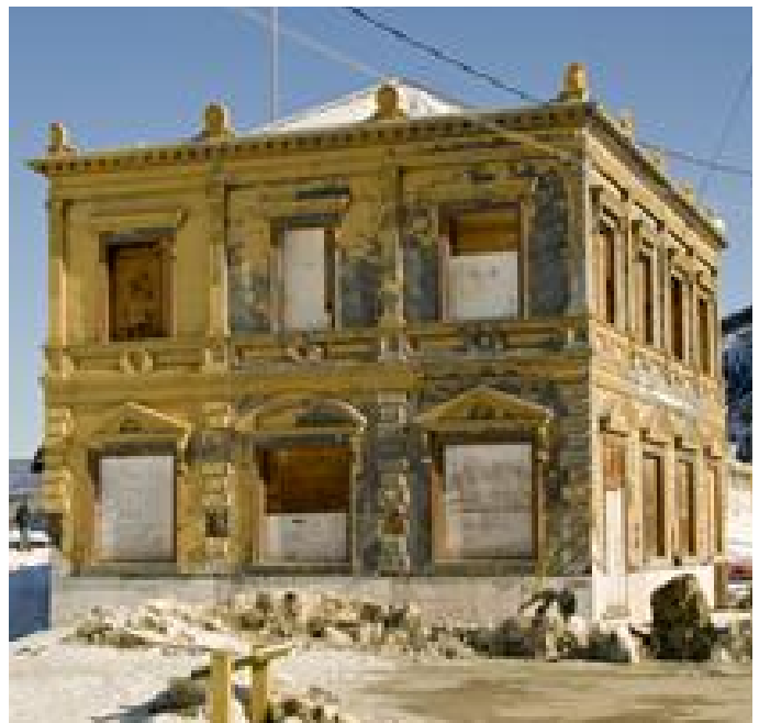
Bank of Commerce Building
